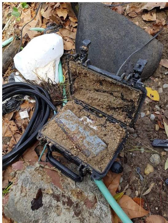
Figure 18: Coffret Tuner Bugadières
